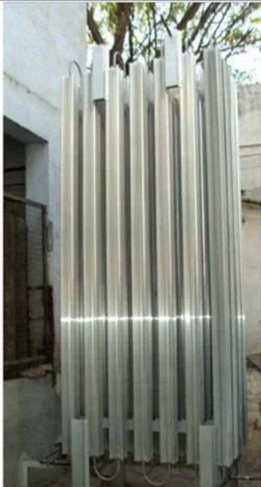
Carbon Dioxide Vaporizer
